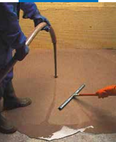
Application of Ultraplan with pump and squeegee
