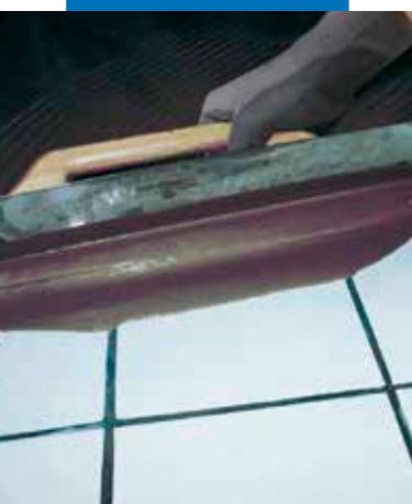
Application of Ultraplan with a metal trowel on an existing ceramic tile floor after the application of Eco Prim T Plus
